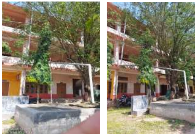
Fig. 4.2 : Rainwater Harvesting System
